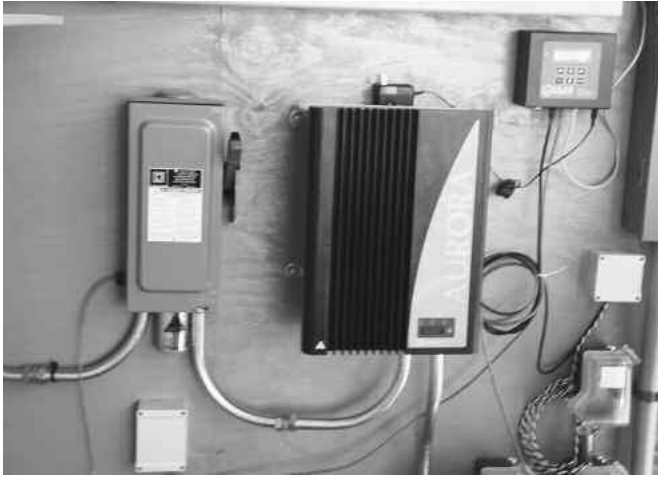
Fig. 8.1: Grid-Connected Inverter. This inverter by Magnetek is designed for batteryless grid-connected PV systems.
