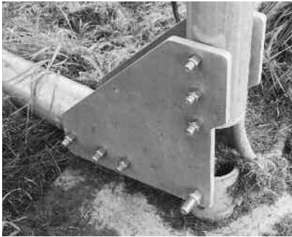
Fig. 6.11: Hinged Base of a Guyed Tilt-Up Tower. The hinge at the base of this tilt-up tower allows it to be tilted up and down to maintain and service the wind turbine.
