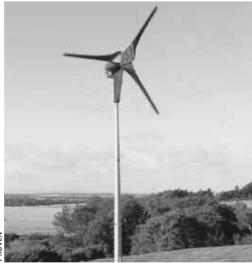
Fig. 6.3: Monopole Tower. Monopole towers are sturdy, well-anchored by a solid foundation, but extremely costly for reasons explained in the text.
