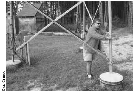
Fig. 5.10: Cable Winch on Tower. Clay Sterling, MREA's Education Director, shuts down a Jacobs wind turbine by tightening the cable attached to the tail of the turbine.
