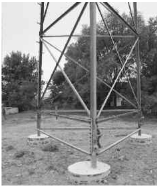
Fig. 6.2a and 6.2b: Lattice Tower . Freestanding lattice towers are made of (a) heavy-duty angle iron, as in this tower erected at the Midwest Renewable Energy Association's headquarters, or (b) tubular steel. Horizontal and vertical bracing made of steel angle iron that runs between the tubular steel legs.
